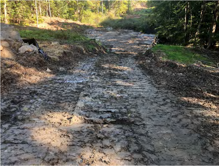
Fig 5: Timber mats at Str's 28 and 29. Viewing north. (9-13-19).
