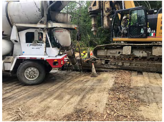
Fig 2: Cement pouring at Str. 106, viewing south. (9-12-19)
