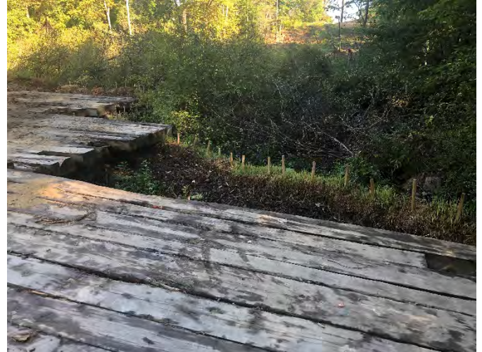
Fig 6: Sediment controls adjacent to the Oyster River and Str. 28. Viewing west. (9-13-19).
