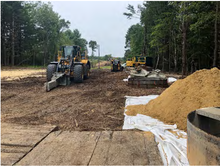
Fig 3: Sand backfill over plastic at Str. 106. Viewing west. (9-12-19).
