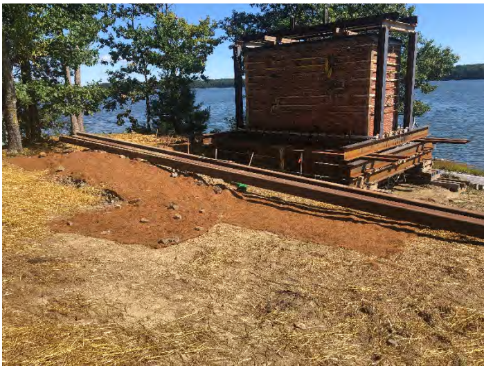
Fig 11: Erosion controls adjacent to the cable house. Viewing east. (9-13-19).
