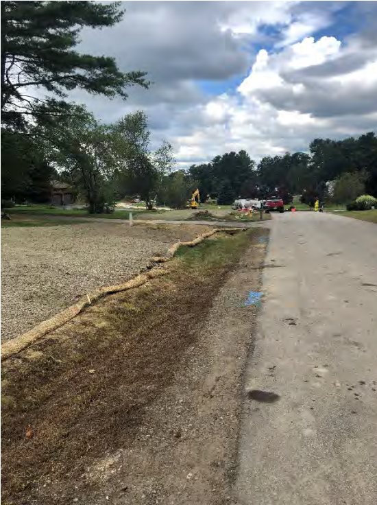
Fig 25: Backfilled trench at Gundalow Landing. Viewing west. (9-17-19).
