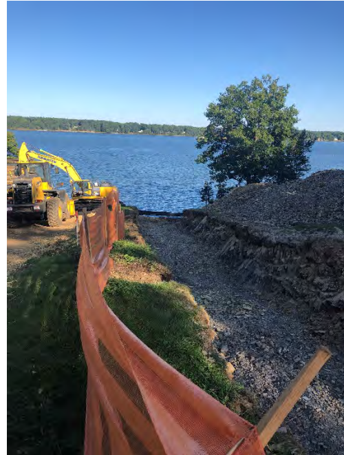
Fig 30: Trenching at Str. 99. Viewing east. (9-18-19).
