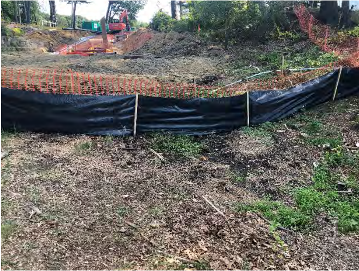
Fig 29: Erosion controls downslope of trench at Str. 99. Viewing east. (9-18-19).
