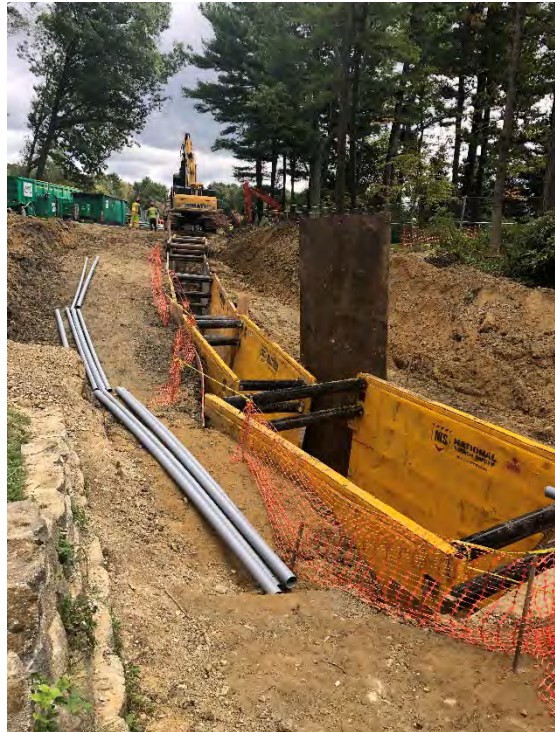
Fig 24: Trenching on the east side of the bay. Viewing northeast. (9-17-19).
