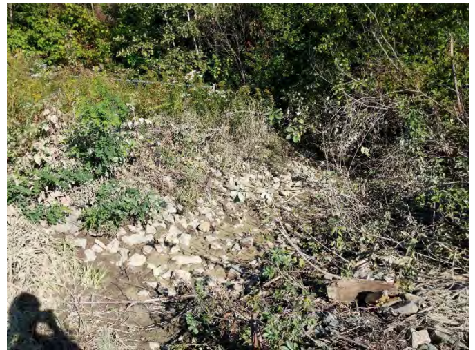
Fig 32: Wetland swale within DW65 following sediment removal. (9-19-19).
