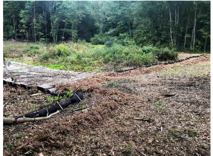
Fig 20: Sediment and erosion controls installed downslope of Str. 107. (9-14-19).
