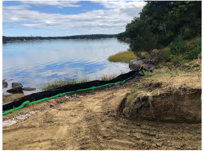
Fig 22: Erosion controls on the west side of the bay. (9-16-19).
