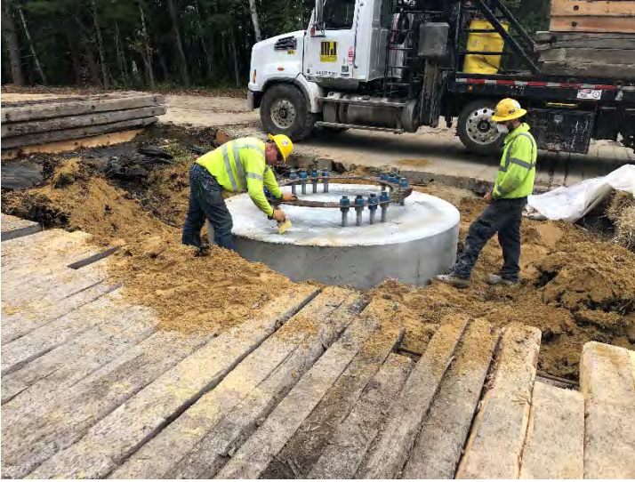
Fig 21: Work at Str. 106. Viewing northwest. (9-14-19).
