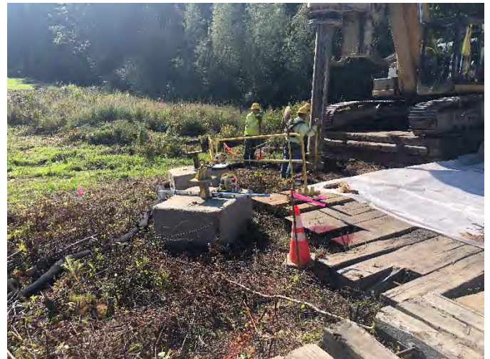
Fig 28: Erosion controls at Str. 112. (9-18-19).
