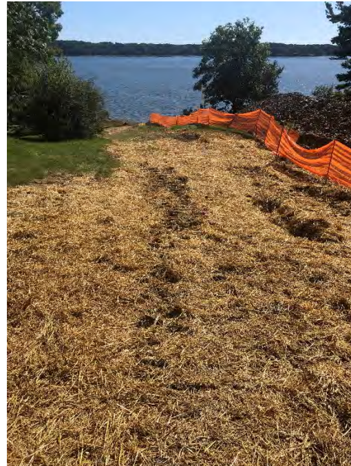
Fig 10: Mulching over disturbed soils on the west side of the Bay. (9-13-19).
