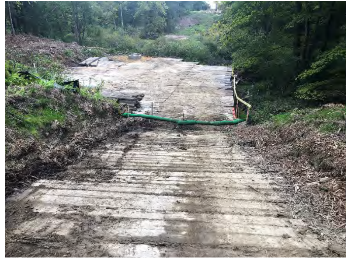
Fig 18: Cleaned up mats looking north towards Str. 28. (9-14-19)
