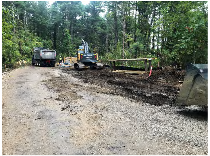
Fig 4: Trench work near Str. 100. Viewing east. (9-12-19).
