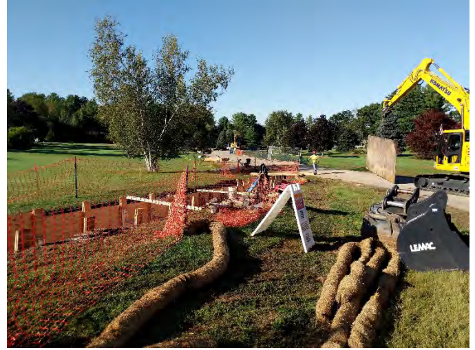
Fig 14: Trenching along Gundalow Landing. Viewing west. (9-13-19).
