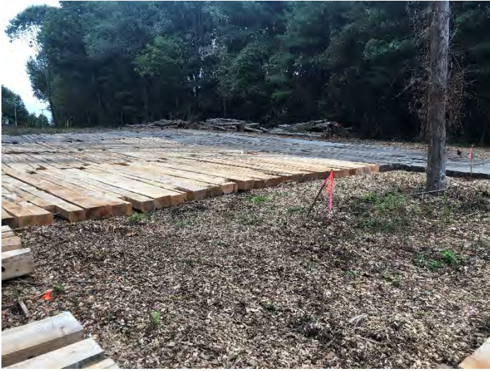
Fig 1: Mat placement at Str. 107, viewing west (9-12-19).
