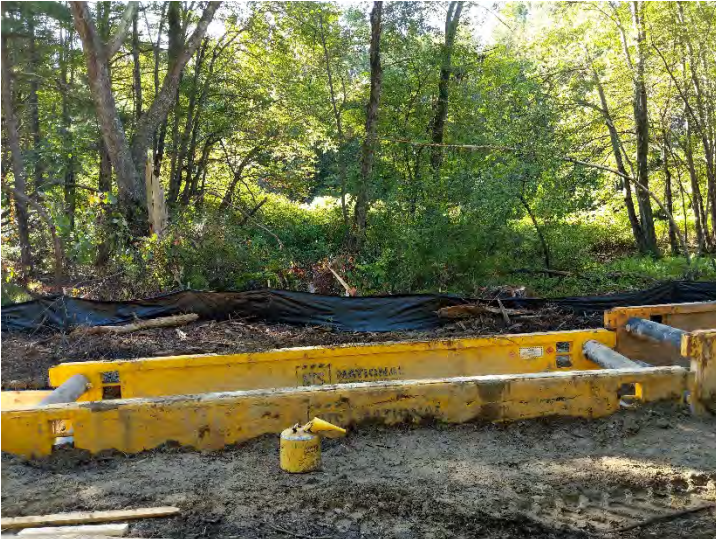
Fig 15: Silt fence along trenching near Str.100 access road south.). Viewing South. (9-13-19).
