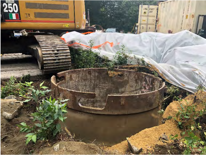
Fig 17: Stabilized Str.31 adjacent to stonewall. (9-14-19).
